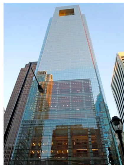
Comcast Center is the tallest building in PA, located in Center City.
